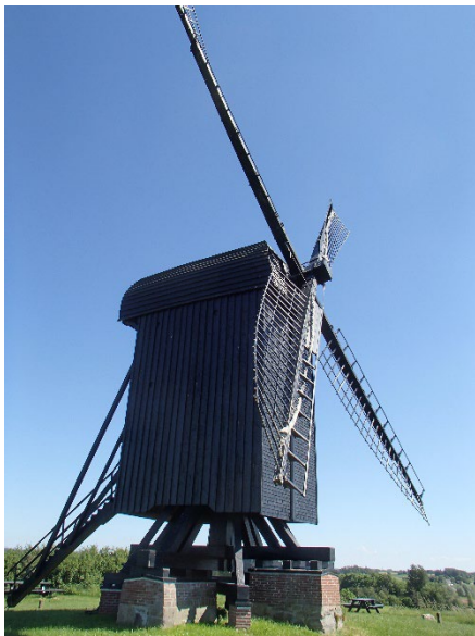
Pipe mill – a stump mill
